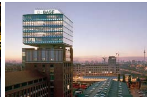
Oberbaum City in Berlin: A leading property site and home of BASF Services Europe GmbH
