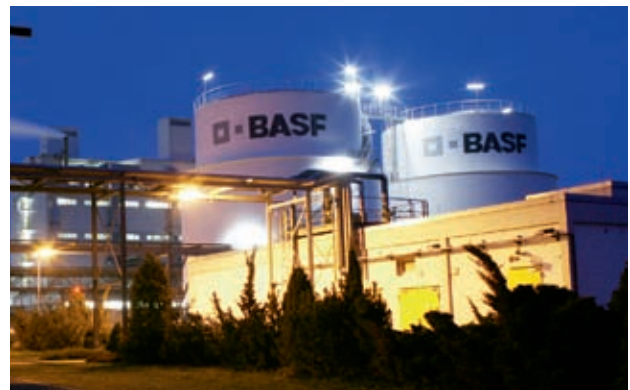
Plant view of the BASF Schwarzheide GmbH in Schwarzheide
